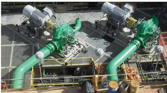
Brazil Refinery Cooling Tower Service
