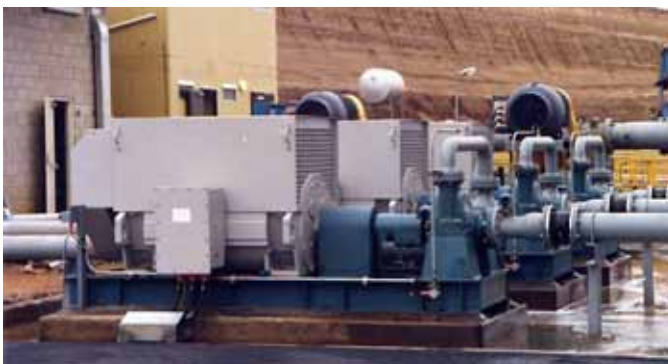
Gold Tailings Pumps in Australia - 3700 4x6-19
