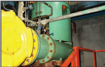
Fairbanks Morse - 50 year old obsolete pump replaced and performance restored. No expensive modifications to piping or foundations required.
