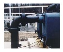
In this installation, two 3" Trash Hogs are being used to control the level of the liquid in these settling ponds. Liquid level controls in the sump determine whether either or both pumps are needed to maintain proper pond level. Trash Hogs were chosen due to their reliable priming capabilities.
